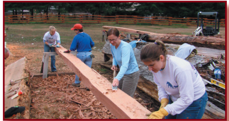
Students apply finishing touches to floor joist for Gilbert's Cabin
