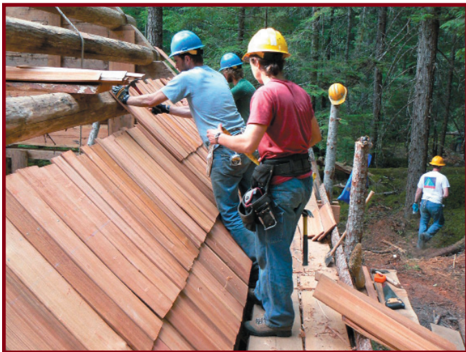
Nailing hand-split shakes to Meadow Cabin purlins
