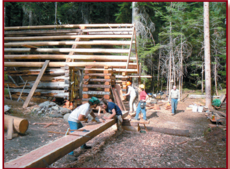
Log preparation and shake splitting at Meadow Cabin
